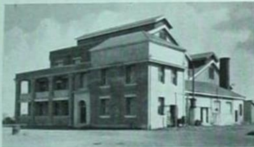
Inkerman Irrigation Power House, Nth. Queensland.
