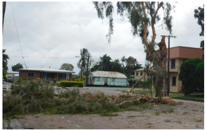
A tree in Seventh Street brought down a power line servicing the area
