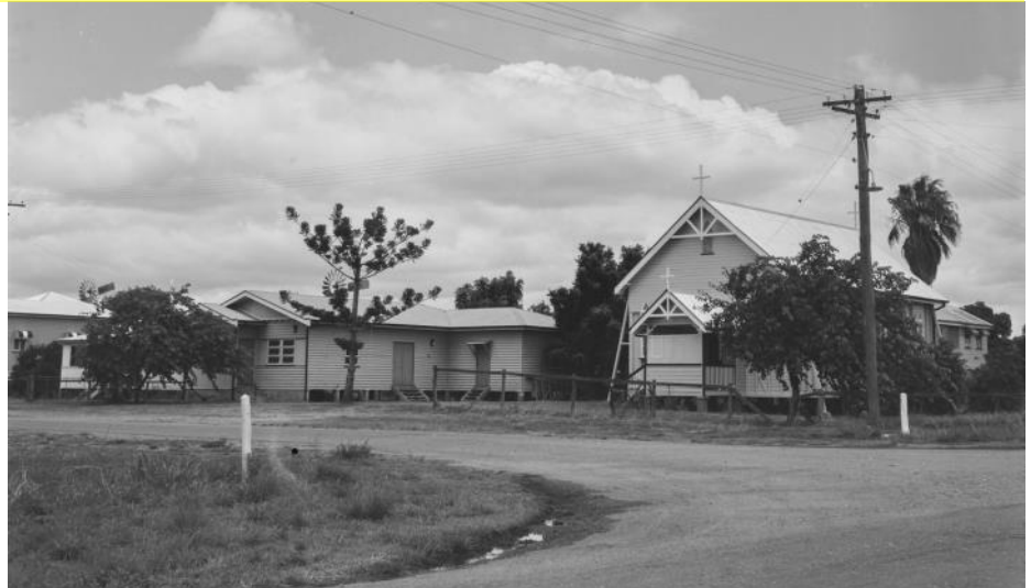
The original St Helen's Anglican Church with the Church Hall before the construction of the current church on the same site
